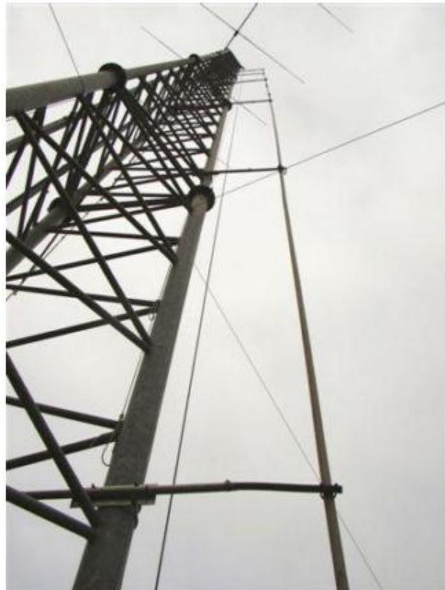
I installed on the side of the tower an aluminium tube of 28 mm. diameter and 20 m. long, with mounting clamps adjustable for both distance and tapping positions.
